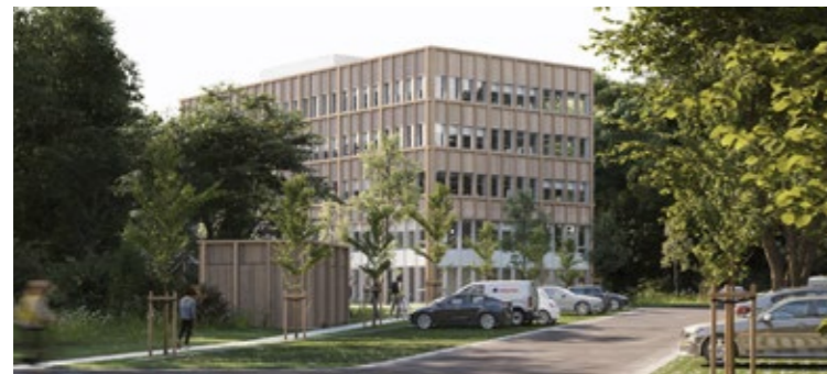
Training centre in Rennes.
